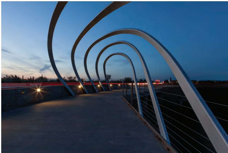
Fig. 1-11. Pedestrian bridge (courtesy of AISC Bender/Roller Committee).
