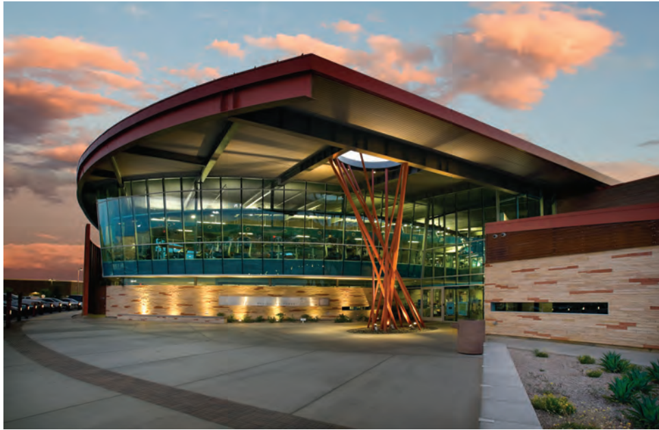
Fig. 1-4. Horizontally curved roof beams for a recreation center (courtesy of AISC Bender/Roller Committee).
