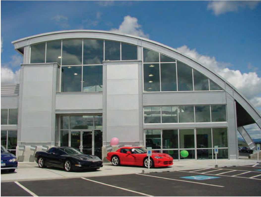
Fig. 1-2. Vertically curved roof for a car dealership (courtesy of AISC Bender/Roller Committee).
