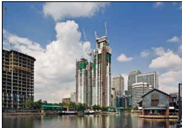
Figure 6.1 High-rise construction. Photo: Laing O'Rourke Plc.
