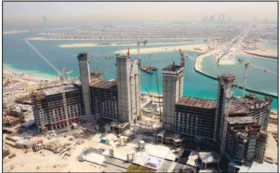
Figure 6.4 An example of a slip-formed core Photo: Laing O'Rourke Plc.
