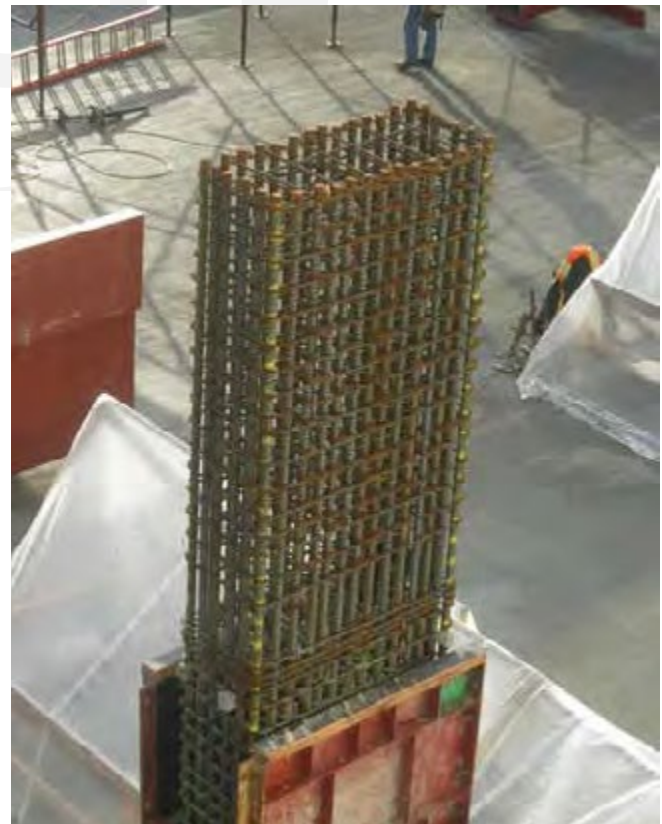
Fig. 2: A column cage with many large vertical bars and cross-ties can be stable enough to eliminate the need for temporary bracing
