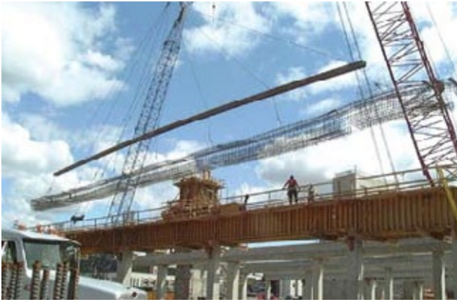
Fig. 5: A multiple-bay, preassembled reinforcing cage can minimize the amount of work that must be done “in the air” and decrease the time required to install reinforcing steel
