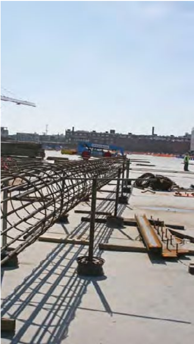
Fig. 4: Horses are used to support a column cage during fabrication
