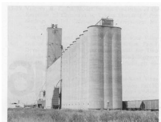
Fig. 16-1 Grain elevator- group of hexagonal and circular silos, Denver, Colorado. (Courtesy of Cargill, Inc.)
